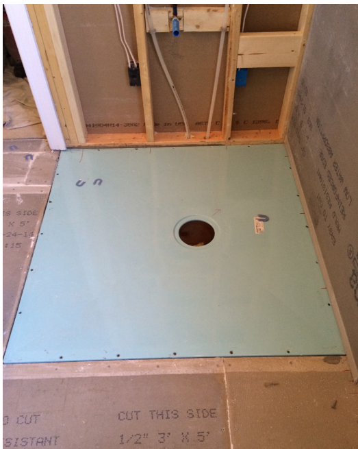
Classic shower base installed on joists.
